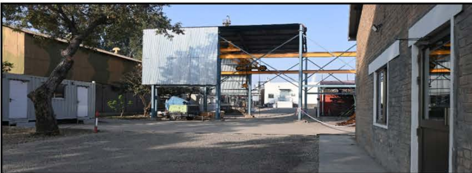
Shed structure & functional Overhead mechanical crane 10 Ton.
